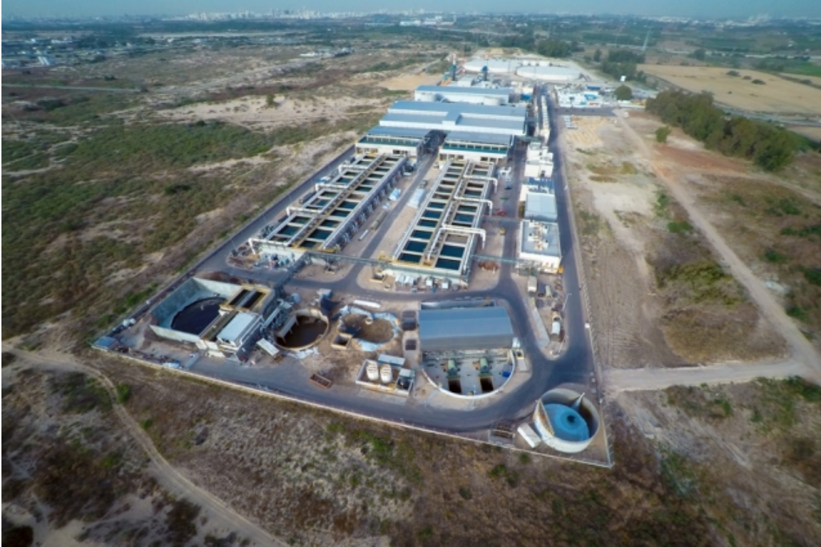
Figure 5.3: The Sorek desalination plant
